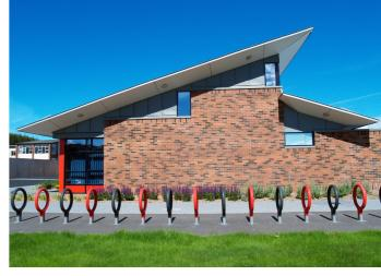
The roofs have been designed to provide clearstorey light into the circulation areas and give deep daylight penetration into classrooms. Each classroom has a section of floor to ceiling glazed screens giving physical and visual links to external play space.
